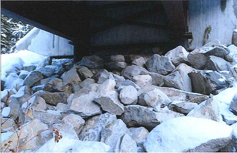
CK2362 Right abutment
