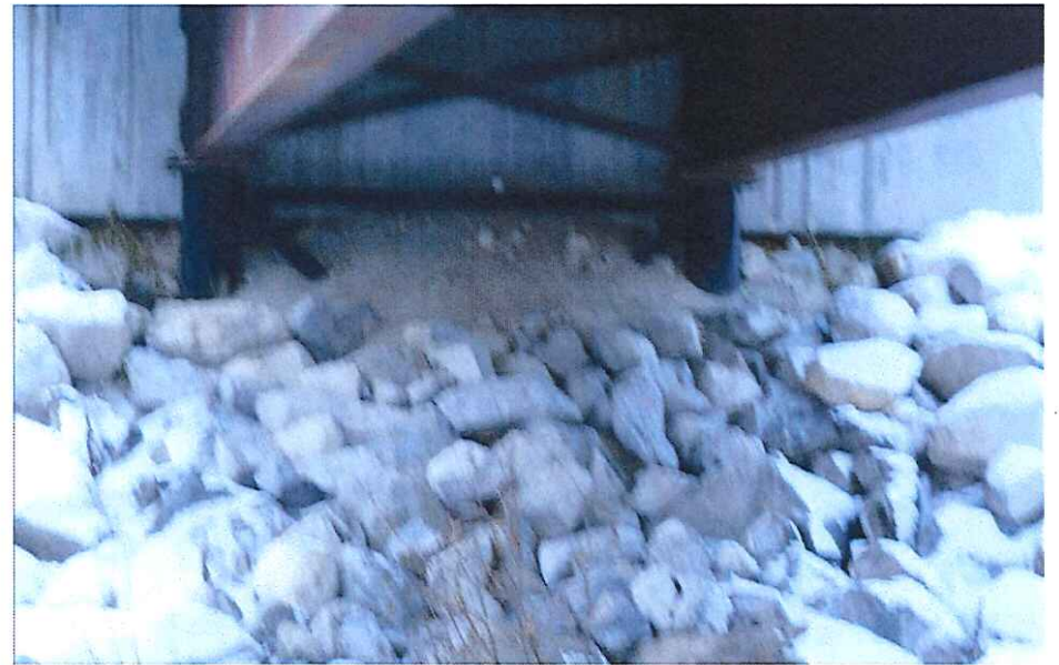
CK2362 Left abutment
